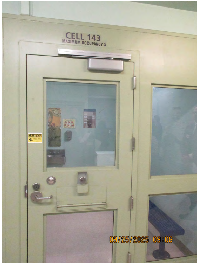
Figure 27. Intake Cell at Mesa Verde
