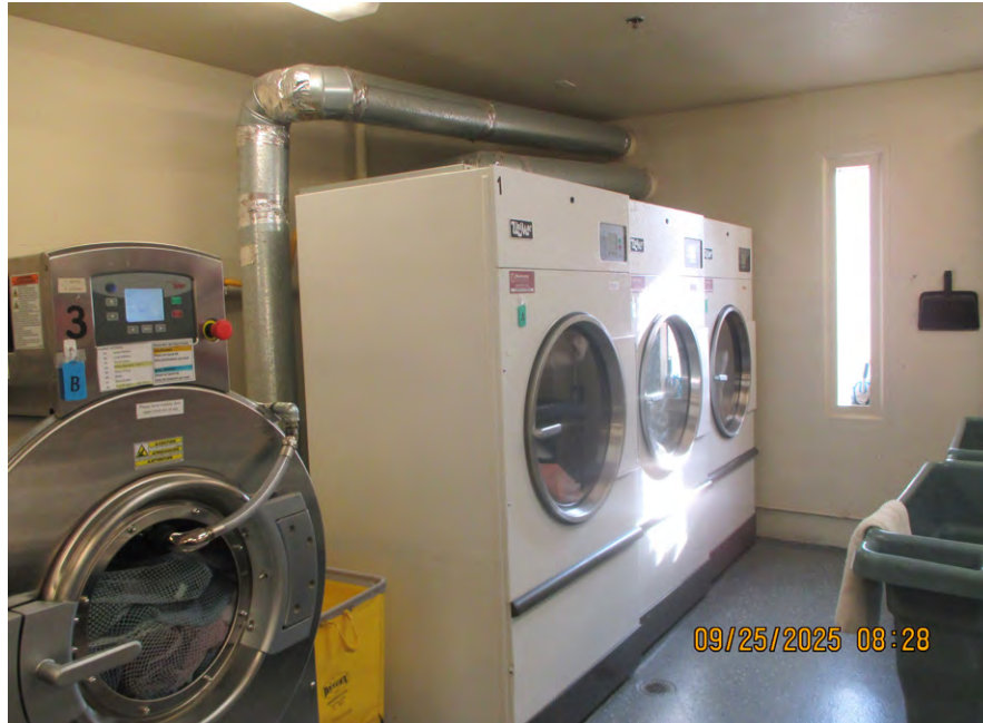
Figure 30. Laundry Facility at Mesa Verde
