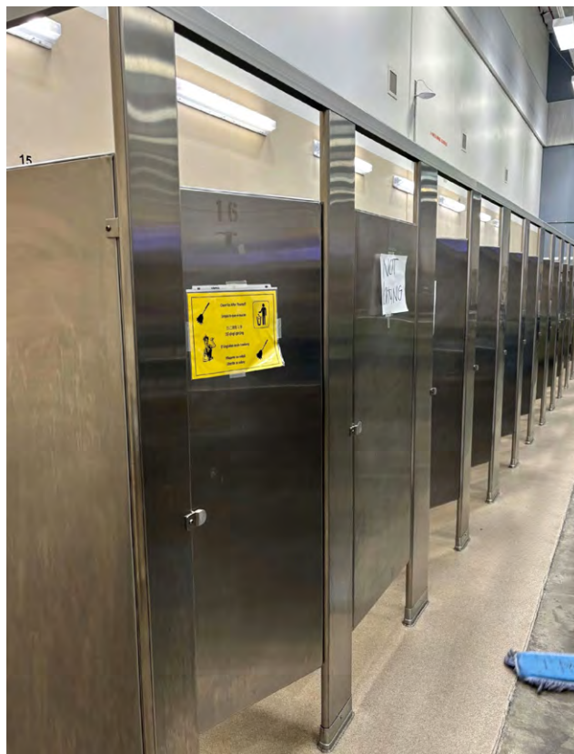
Figure 51. Doors to Toilet in Housing Unit at Otay Mesa
