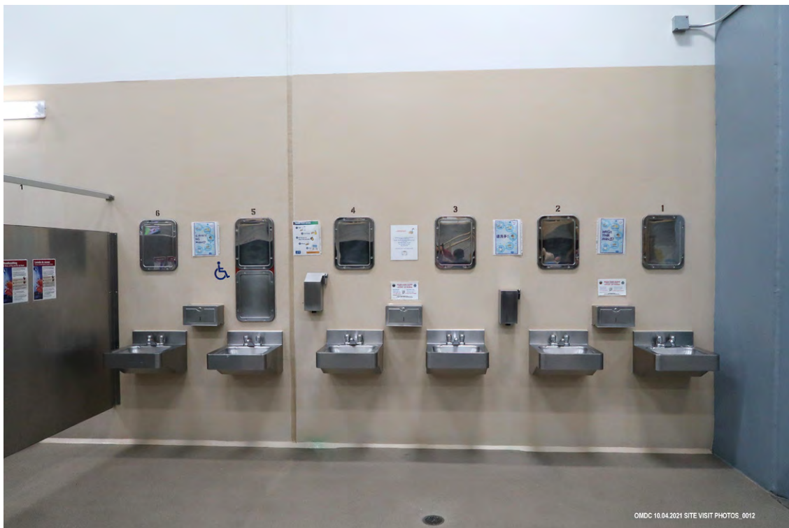
Figure 50. Sinks in Housing Unit at Otay Mesa
