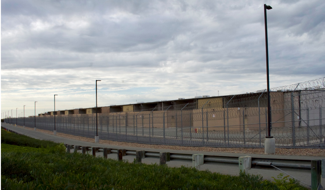
Figure 54. Exterior Walls of Housing Units' Outdoor Recreation Areas at Otay Mesa
