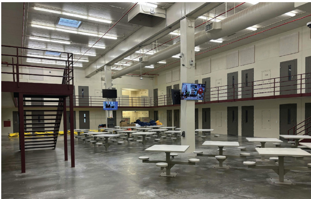
Figure 61. Housing Unit at Cal City
