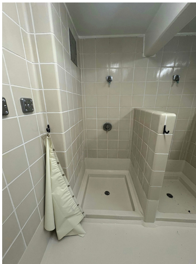
Figure 62. Shower Facilities at Cal City
