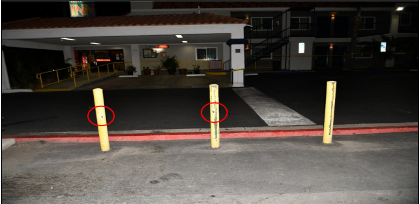
Two bullet strike marks on the parking bollards
