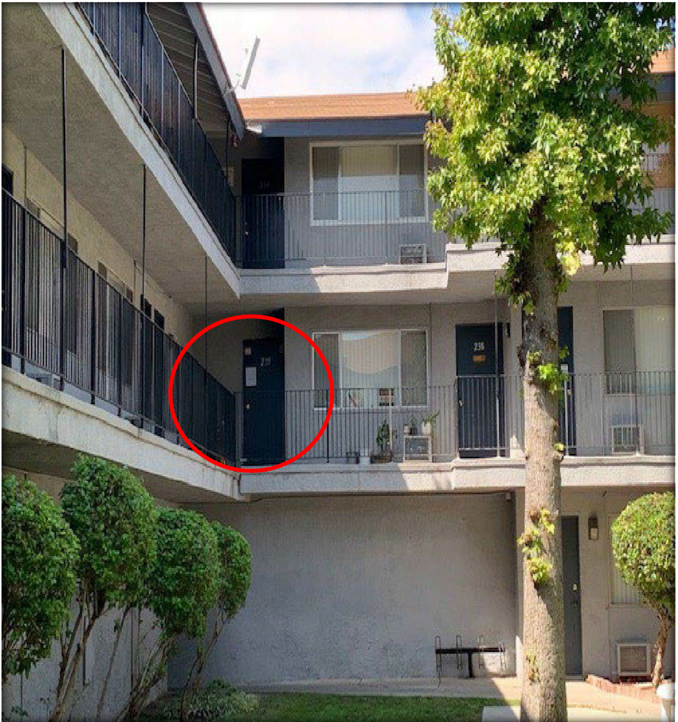
Figure 5 – Unit #239 as seen from unit #126 (first floor)
