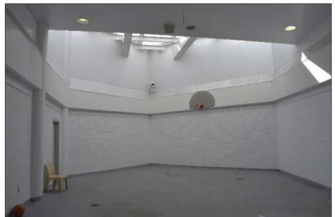
Figure 26. Photo of Recreation Area in Modular Housing
